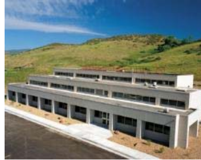
NREL Thermal Test Facility 10,000 ft 2 (929 m 2 ) mixed office/light laboratory building in Golden, CO.
