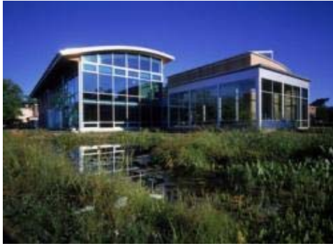
Adam Joseph Lewis Center for Environmental Studies , Oberlin College 13,600 ft 2 college building located in Oberlin, OH.
